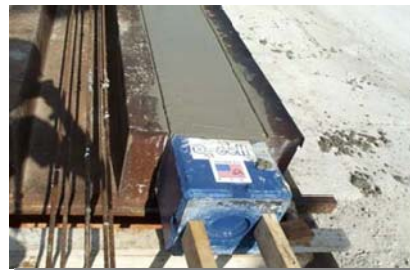
300x300mm O-cell concreted
